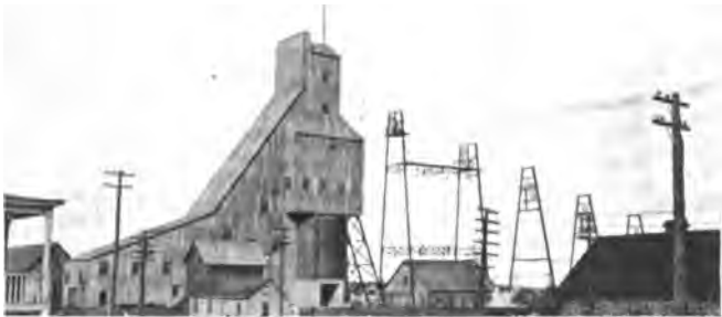
B. ROCK HOUSE AT SHAFT NO. 2, QUINCY MINE.
